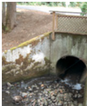
Culvert replacement is key to fish habitat restoration.
